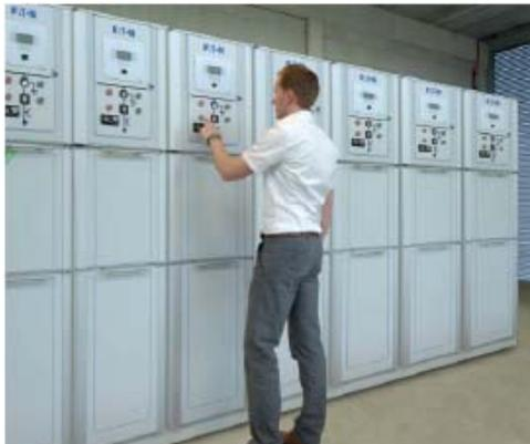
Figure 3. State of the art, fixed medium voltage switchgear
